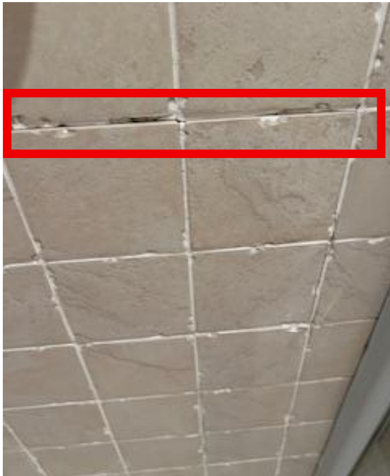
Shower room above, tiles in places need regrouting. These are set onto a plasterboard wall, and the reverse side is damp. Re grout and intrusive investigation
