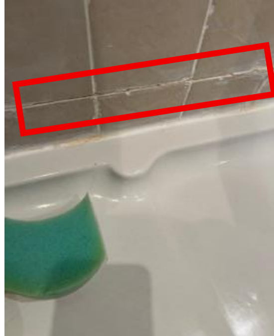
Shower room above, tiles in places need regrouting. These are set onto a plasterboard wall, and the reverse side is damp. Re grout and intrusive investigation
