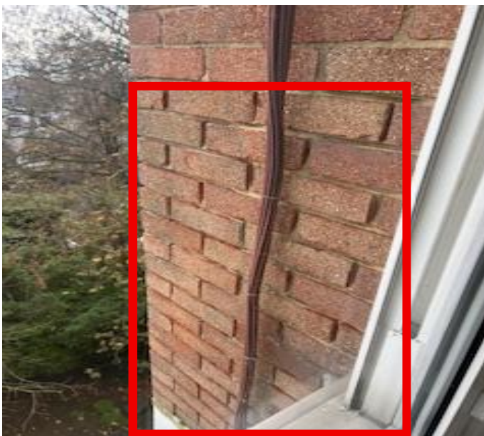
View from bay window, also faces the sea, pointing has been raked out, above
