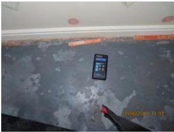
Concrete floor, wet and damp proof membrane, is suspected as faulty
