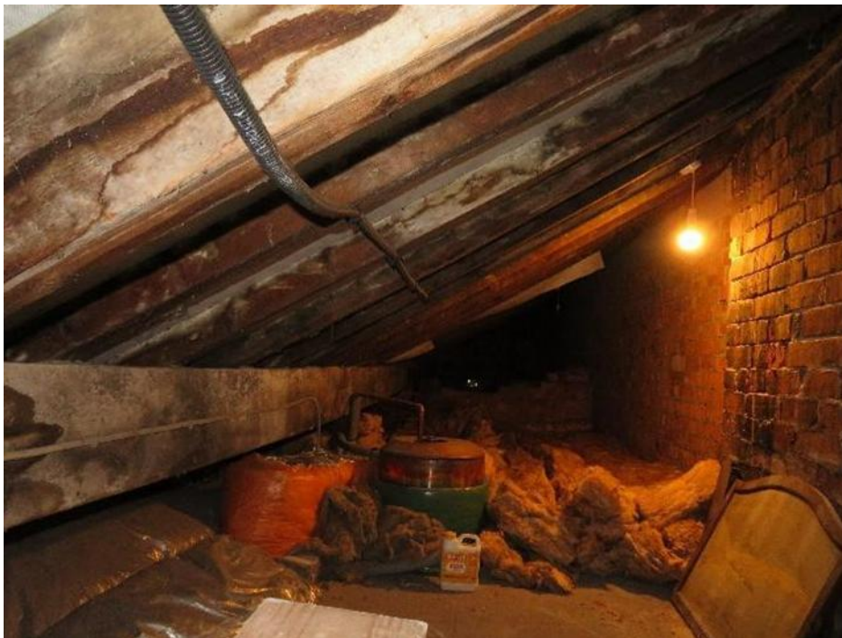
Visible presumed mould and water staining
